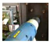
3. Remove the mounting plate. Drill 3/4" hole from front through the pilot hole.
