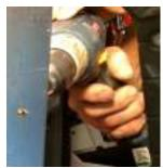
9. Insert the locking screw and secure it with a hex nut. Bend the cam slightly to the front or back to ensure a tight fit over the screw when closed.
